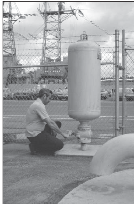
Refineries — Shock from pump starting and stopping
