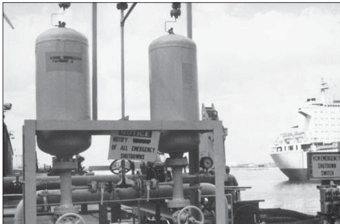
Liquid bulk handling absorbs surges and shocks from fluids in motion
