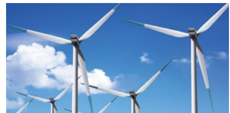
Wind turbine speed monitoring
