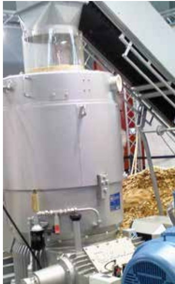
Level control of wood chips
